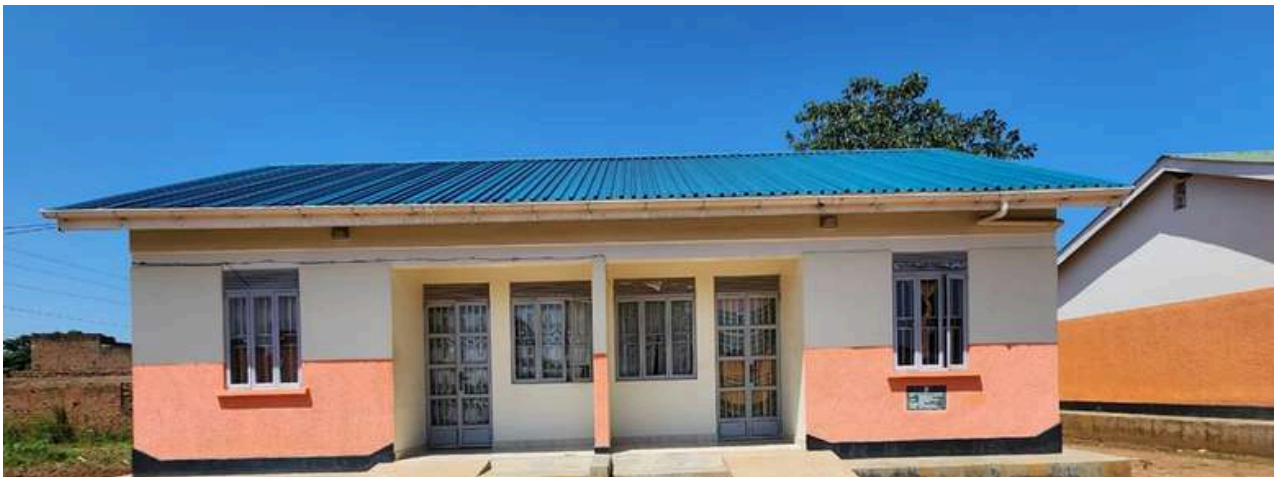
Staff twin house constructed at AWEI HC III in Alebtong district
